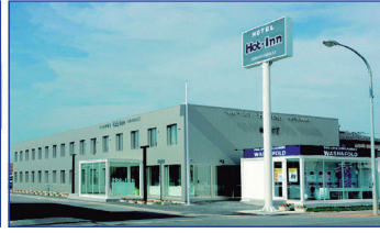
Modular Container Hotel
