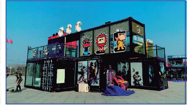
Modular Container Town
